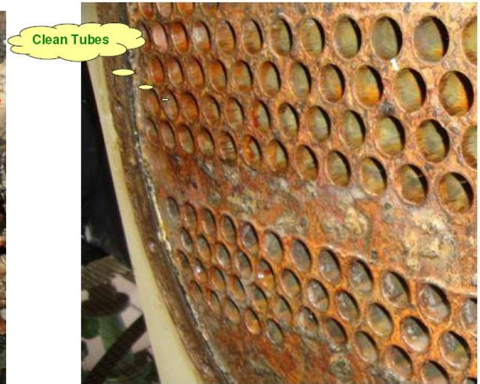
Tubes After ATCS Installation
