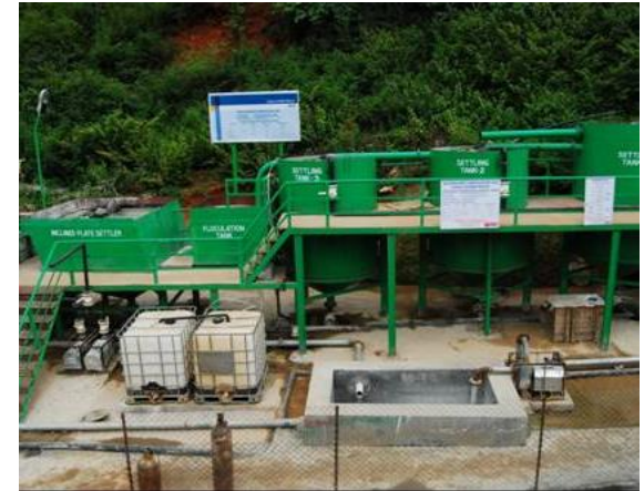
WTP at Vizag Cavern
