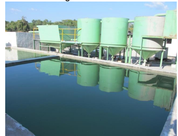
WTP at Padur Cavern
